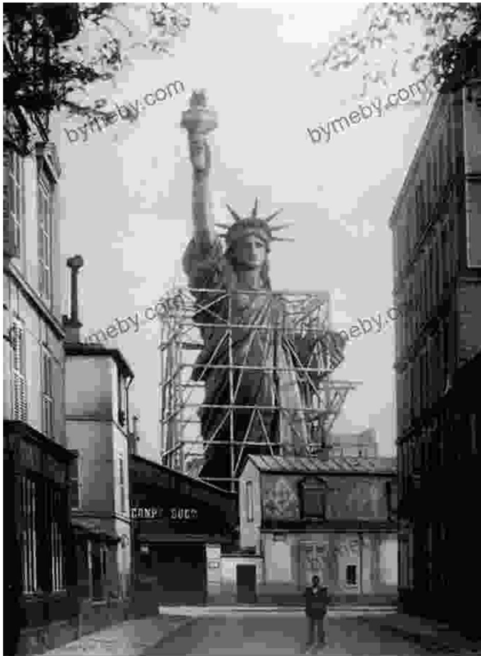
Bartholdi meticulously crafted a clay model of the statue, which was then used to create a series of plaster casts. These casts served as templates for the copper sheets that were hammered into shape to form the statue's exterior. The process of assembling the statue in Paris was a monumental undertaking, requiring the coordinated efforts of hundreds of skilled craftsmen.
